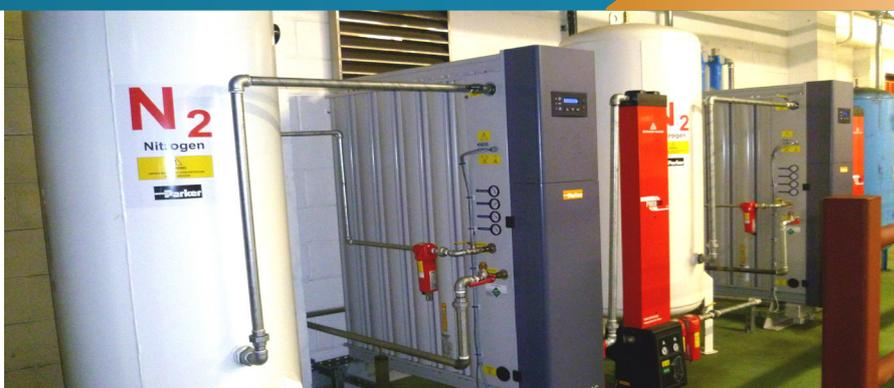
MAXIGAS Nitrogen Gas Generators produce nitrogen gas from compressed air and offer a cost-effective, reliable and safe alternative to traditional nitrogen gas supplies such as cylinder or liquid.
